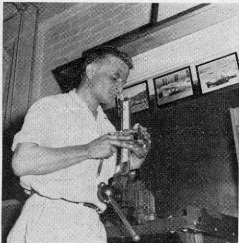
2 (opposite page) After installation, and with engine running, throttle stop is adjusted until water manometer reads .50 at about 3000 engine rpm.
